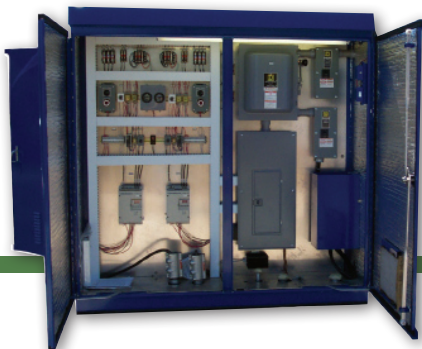
Outside Duplex Pump Control Panel
